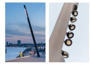
Poles are mounted at intervals of between 18 and 40m at heights of 6.5 m or 8.5m, with each pole assigned to a staircase, to which it is tilted at an incline of around 15°.
