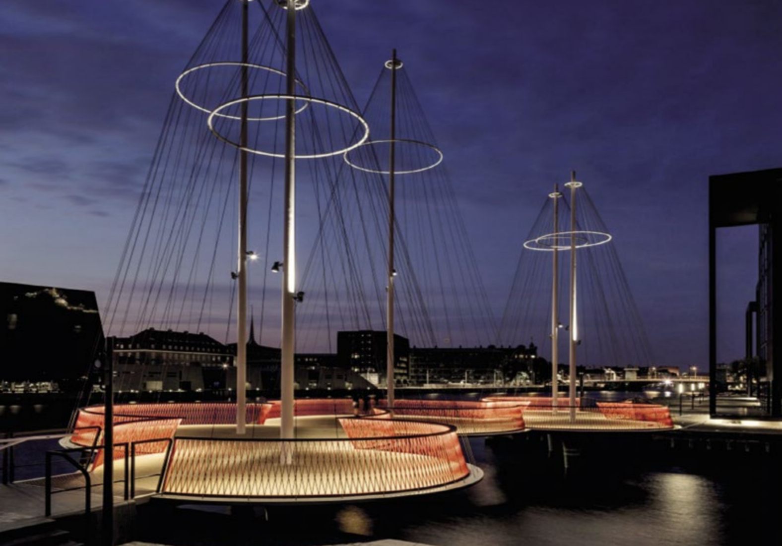
Circlebroen (Circle Bridge), Copenhagen, Denmark - Olafur Eliasson © Anders Sune Berg
