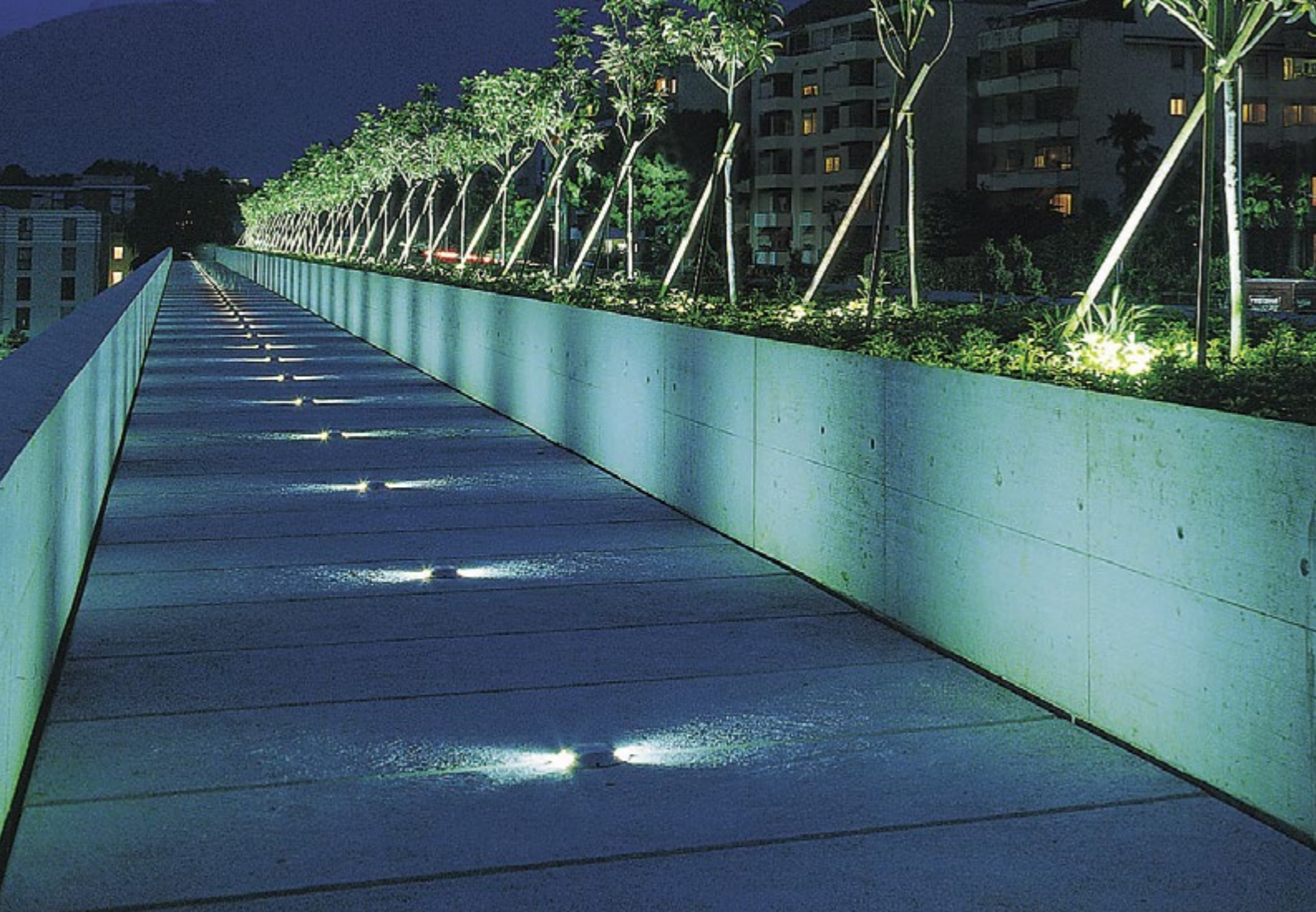
Walkway, Locarno, Switzerland © SIMES S.p.a.
